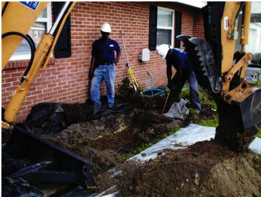
Picture 2: UST 1290Eagle excavation in progress.
