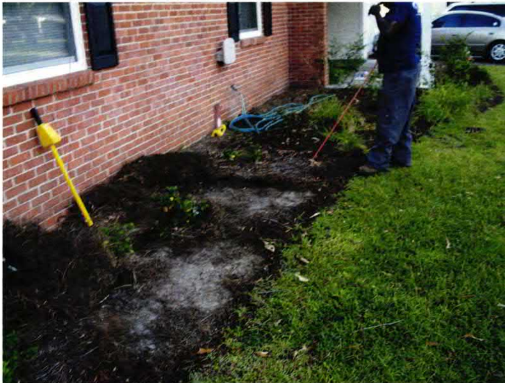
Picture 1: Location of UST 1290Eagle.
